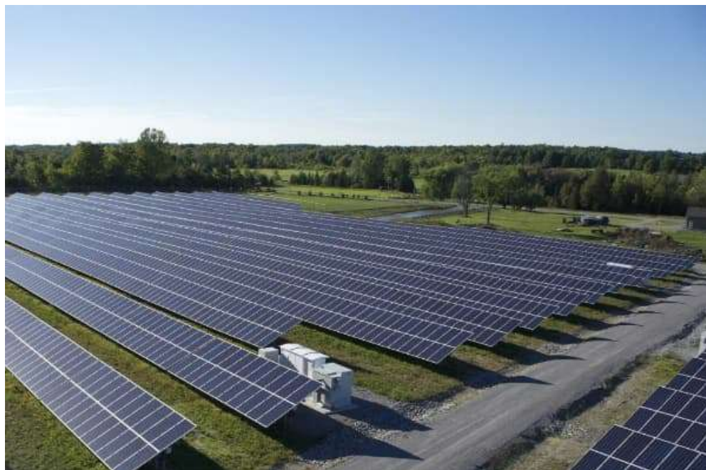
Plate 2 Typical Fixed Solar PV Panels (with Conversion Unit/Inverter)
